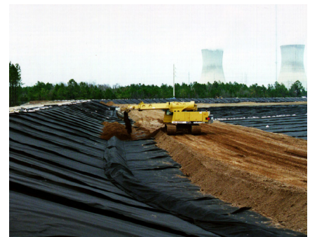
[Cooling Water Pond Storage]
