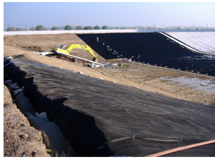
[Geotextile Installation]
